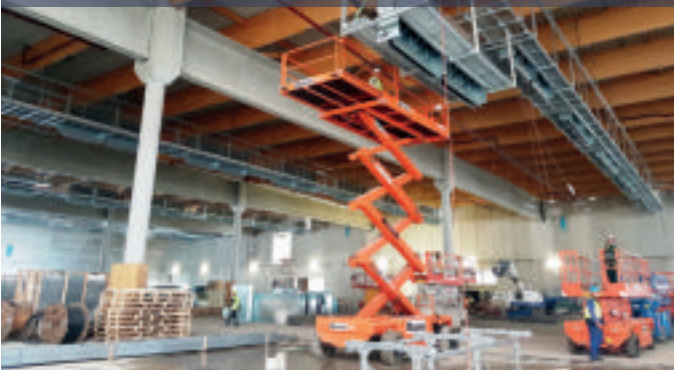
Installation of the siFramo catwalk modules
