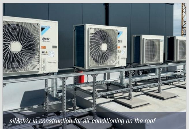
siMetrix connected directly to the steel beam
