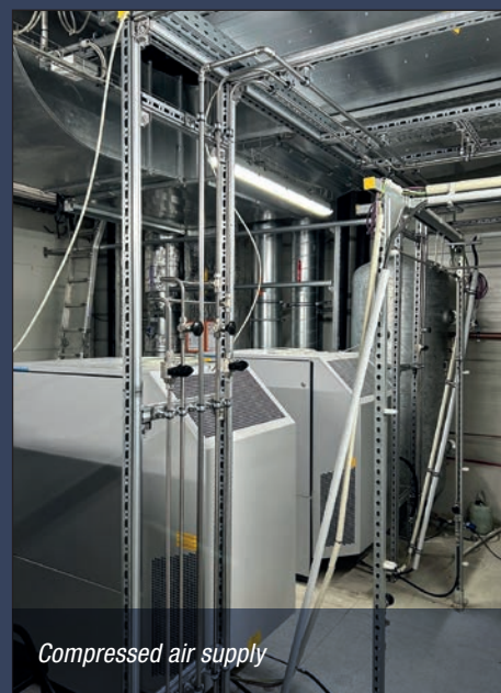
3-dimensional mounting grid for areas with high installation density and when flexibility is required.
