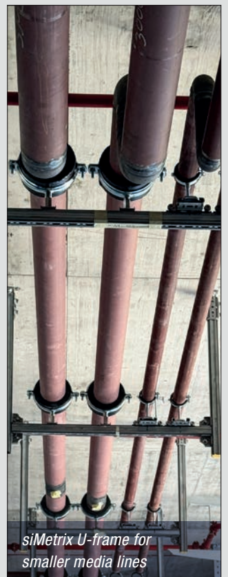
siMetrix connected directly to the steel beam
