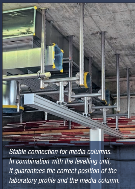
3-dimensional mounting grid for areas with high installation density and when flexibility is required.
