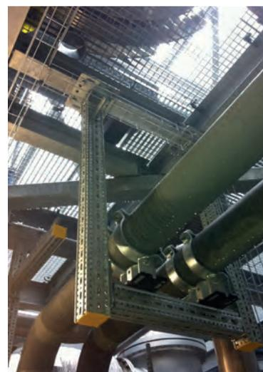
Archive photo: Modular bolted siFramo system for rapid assembly of secondary steel constructions
